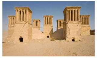
A windcatcher looks like a tall, decorative chimney, usually with two or more open sides. It catches the breeze that blows well above ground level and channels it down into the house below. This displaces warm air that is expelled through the opposite face of the windcatcher. In some designs the incoming air blows over water, providing further cooling. This simple design can reduce the temperature inside a building by 8C to 12C. Even in the complete absence of wind, a
